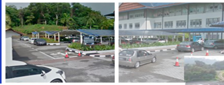
Langkawi Hospital, Malaysia 76 kWp Carpark Solar PV system
