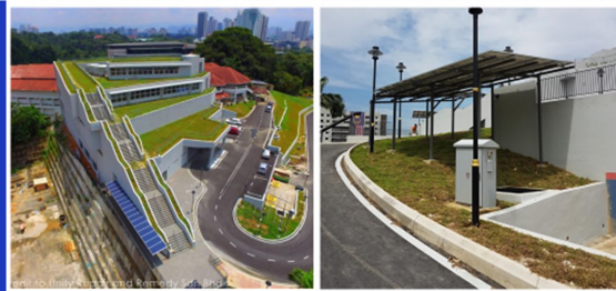
Memorial Tun Hussein Onn, Malaysia 11.2 kWp Side walk Solar PV system
